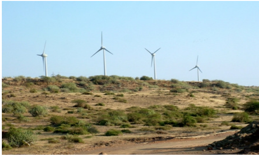
Figure 12: Samana wind farm, the largest wind project at Gujarat
